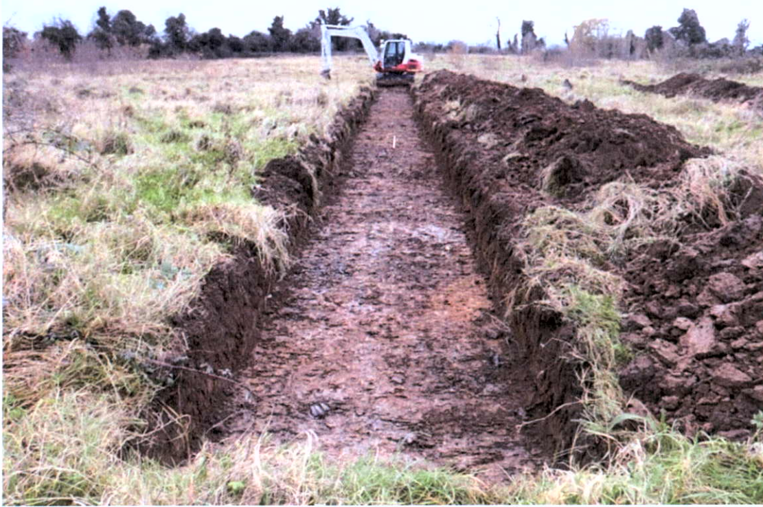
Photograph 12.3 Test Trench 3 from North
