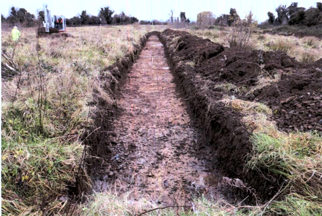
Photograph 12.2 Test Trench 2 from North
