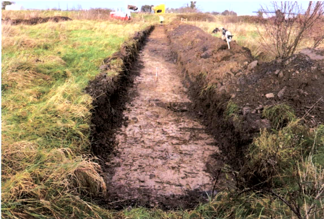
Photograph 12.7 Test Trench 7 from North
