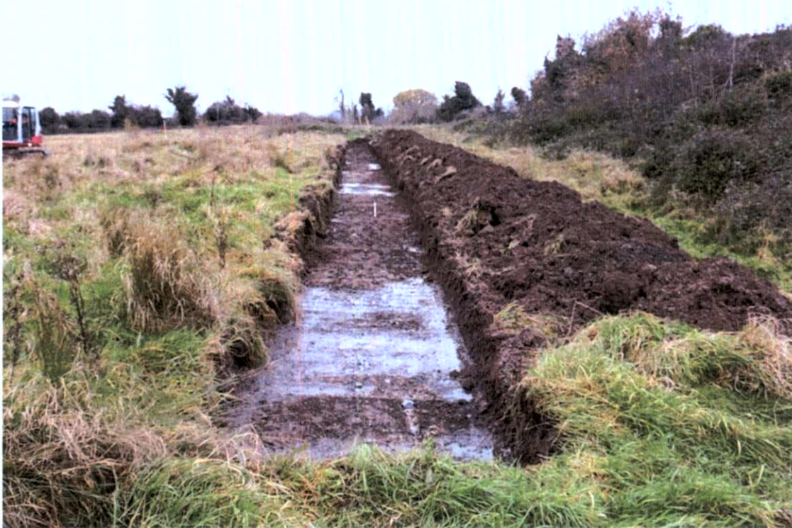
Photograph 12.1 Test Trench 1 from North
